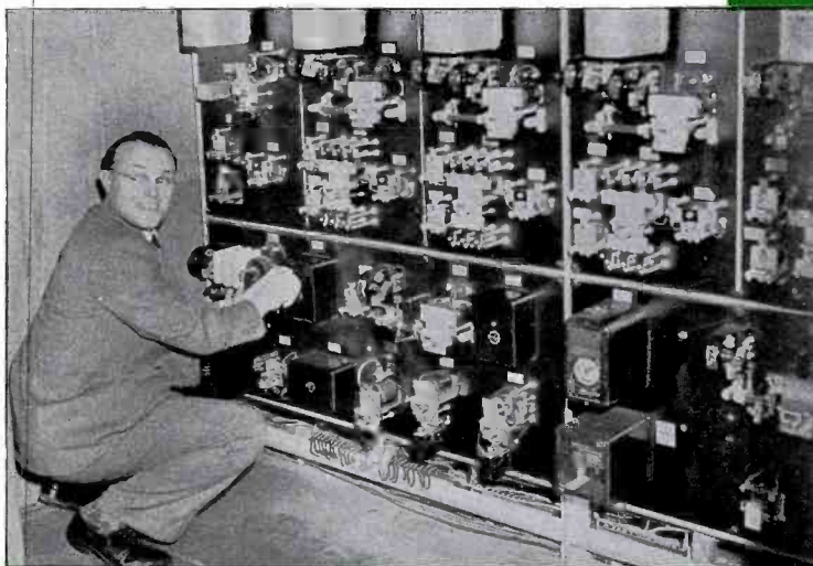
JOE WHITEHOUSE , Chief Transmitter Engineer, makes an adjustment on the largest relay panel ever employed by any commercial radio station in the United States. The relay panel, created in the WLW research laboratory, operates a transmitter from throughout the transmitter.
